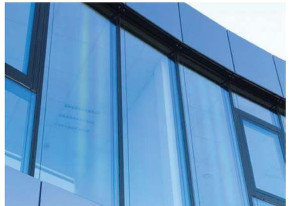
Figure 4: Typical anisotropy phenomena in architectural glazing. The glass pane in the middle of the image has been produced in an isotropy-optimised toughening process and shows no disturbing optical effects (photo courtesy of arcon).
